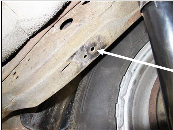
Figure 5 – Left side factory hanger holes
