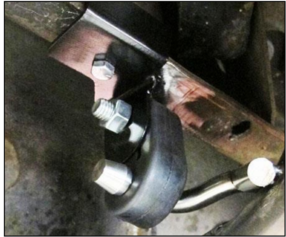
Figure 4 – Right tailpipe hanger bracket
