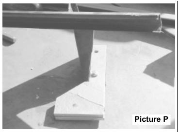
Above picture of bracket s bolted on rear channel.
