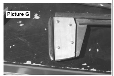
Above picture is of the front of the sash with  $#10 \times 24 \times 3/4$ " bolts installed.
