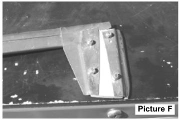
Above picture is of back of sash with nylon lock washers.
