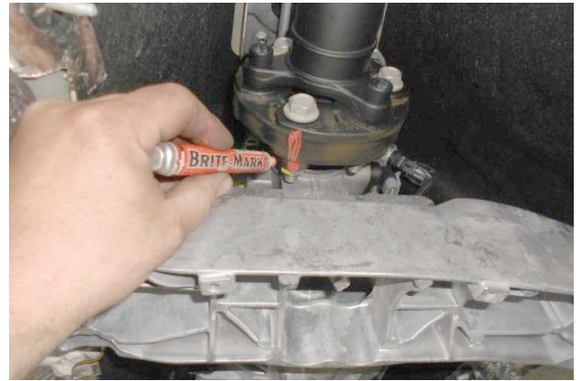
16. To remove drive shaft, begin by making alignment mark on flex coupling and transmission flange.
