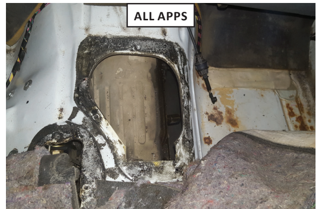
27. Deburr edges and remove loose or excess material from tunnel under where base plate fits.
