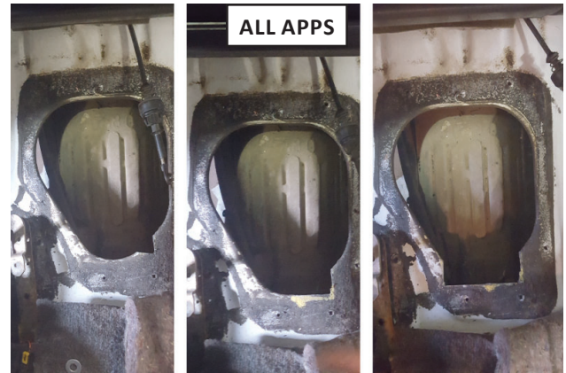
26. Make a cut within marks, compare it to base plate and mark again as necessary. Continue this until base plate fits flat against tunnel.
