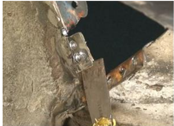
Figure 11b – Removing & Bending Lap Flange
