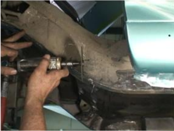
Figure 10a – Mark & Cut Vertical Ends First
