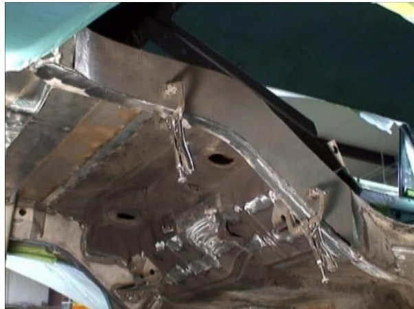
Figure 12 - Fitting and Trimming the New Frame Rail Close Out
