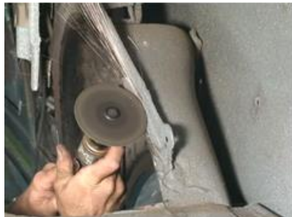
Figure 9b – Cutting the Horizontal Flange
