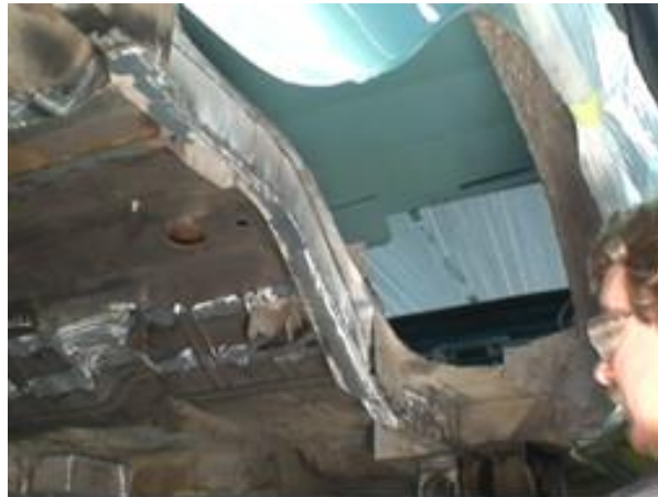
Figure 10c – Finished Frame Rail Clearance
