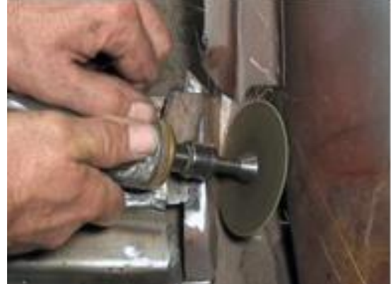
Figure 6b – Removing the Brace
