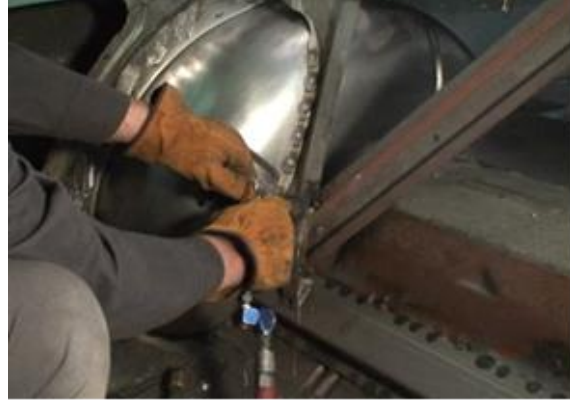
Figure 16b - Welding Modified Brace
