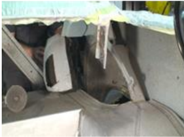
Figure 7c – Removing the Factory Wheel Well
