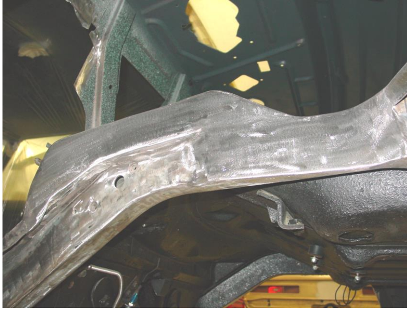
Figure 7 - Framerrail with Closeouts Installed
