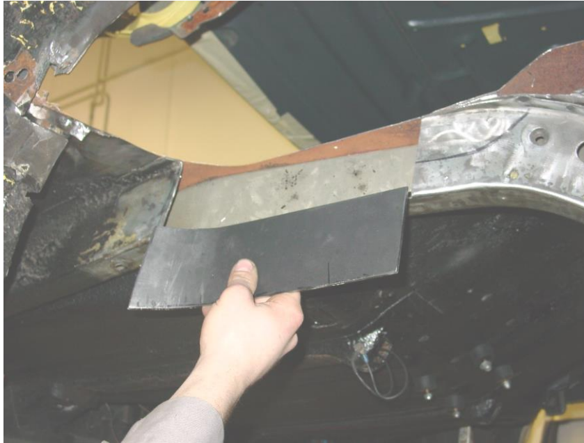
Figure 5 - Frame Rail Closeout
