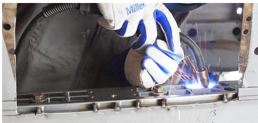
Figure 17 - Finish Weld Adapter Plates & Floating Stanchions
