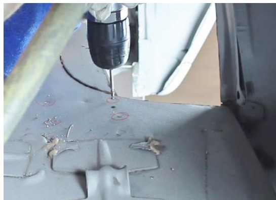
Figure 15 – Drill-Out Spot Welds
