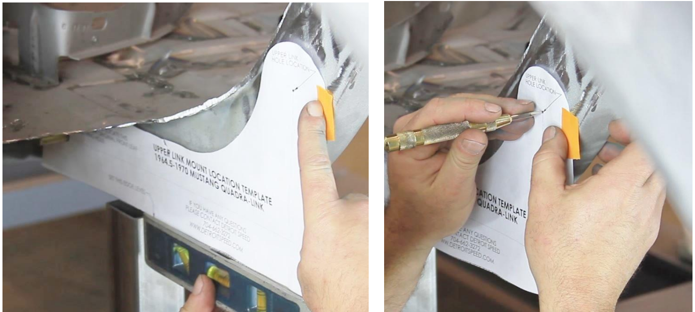
Figure 7 - Upper Link Mount Hole Location
