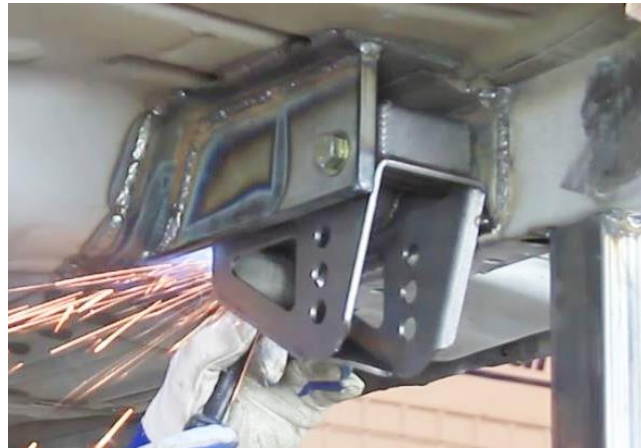
Figure 17 – Weld Front Lower Link Bracket
