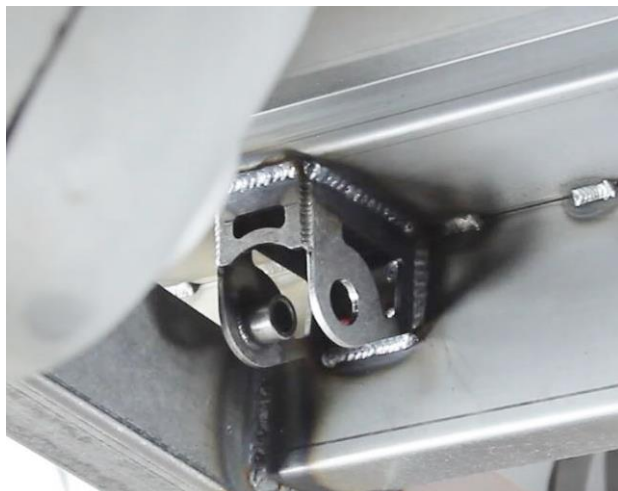
Figure 24 - Weld Upper Shock Mounts
