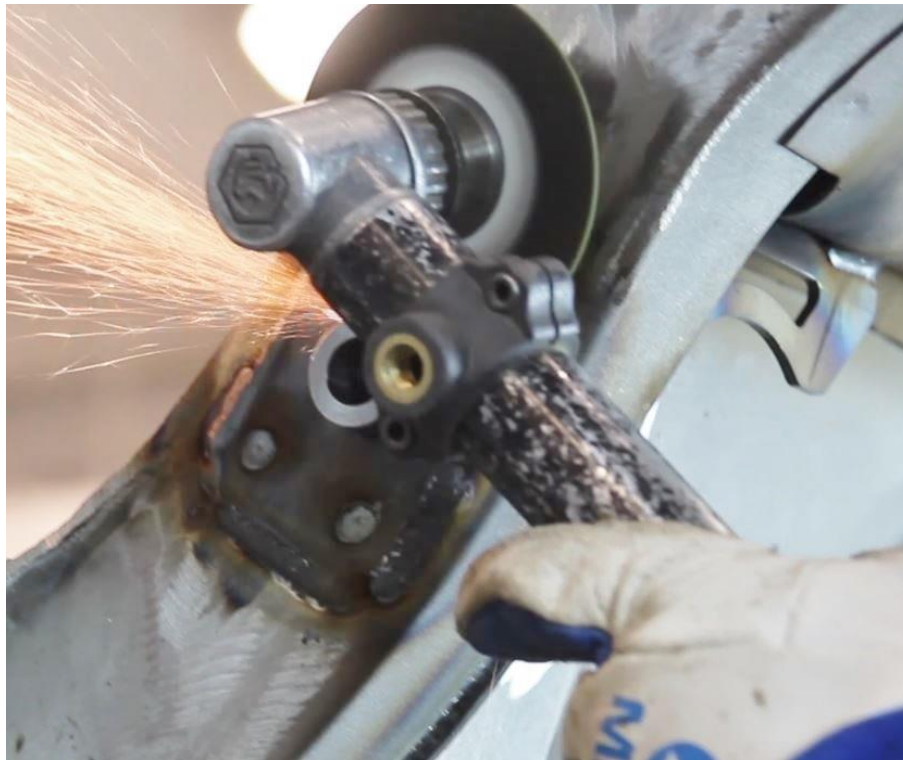
Figure 15 - Cut-Off Crush Tube Flush with Frame Rail
