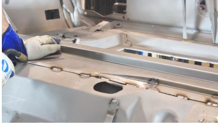
Figure 22 - Stitch Weld Front of Crossmember
