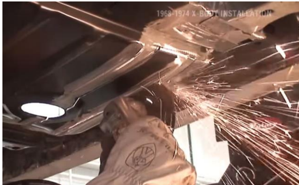
Figure 8 - Cut Floor Pan
