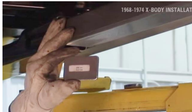
Figure 12 - Tack Weld End Cap in Place
