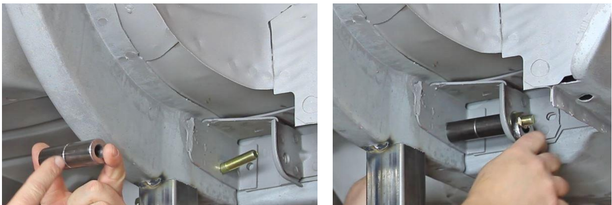
Figure 4 - Install Weld Spacer
