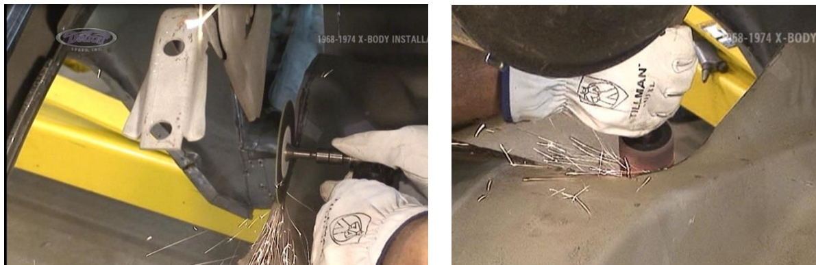
Figure 20 – Finish Cut and Grind Pre-Marked Lines
