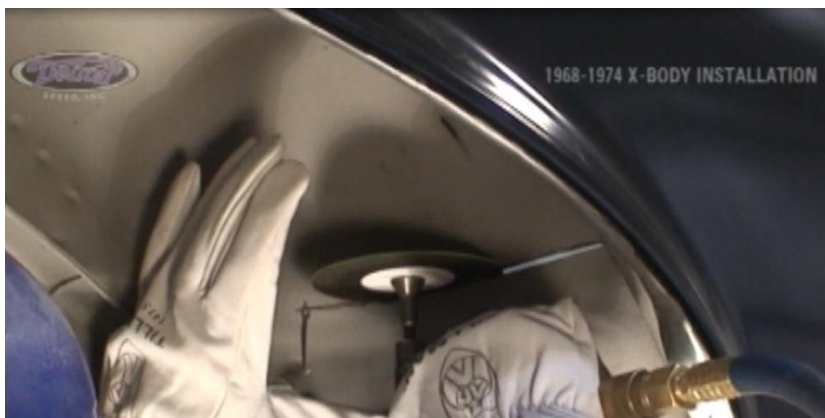
Figure 10 – Start Cutting the Stock Tub
