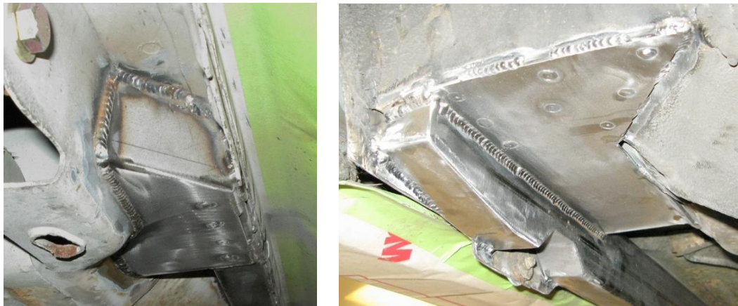
Figure 15 - Finish Weld Doubler & Closeout Plates
