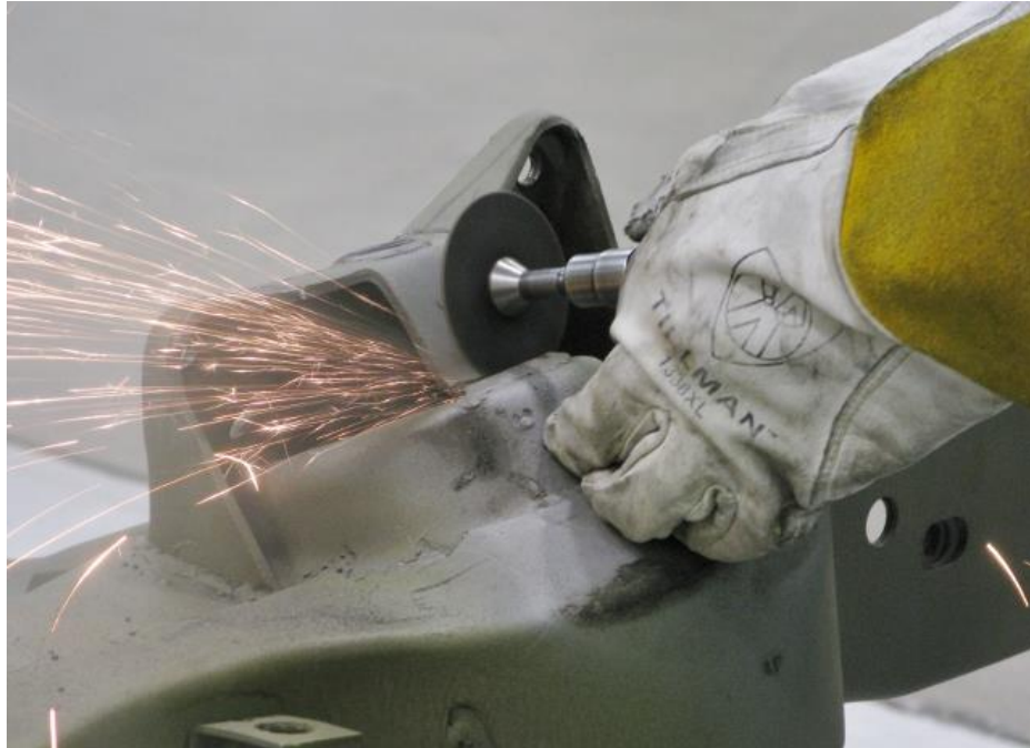
Figure 6 - Cut Factory Upper Shock Mount Bracket
