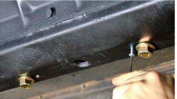
Figure 38 – Install Crossmember Nut Plate
