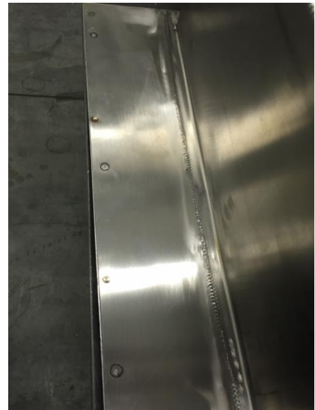
Figure 3 - Verify Hole Location
