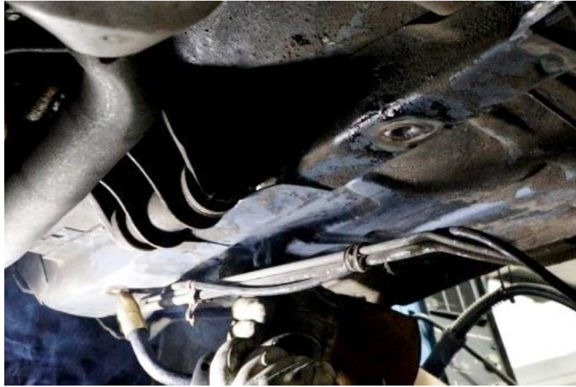
Figure 42 - Weld Front Connector
