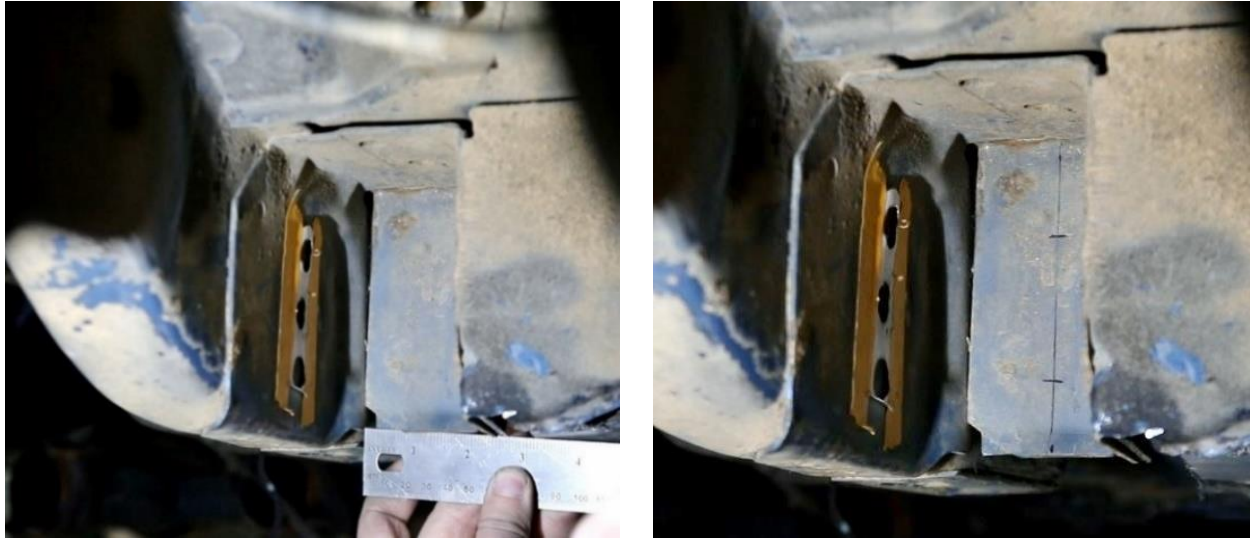
Figure 31 - Locate Plug Weld Holes
