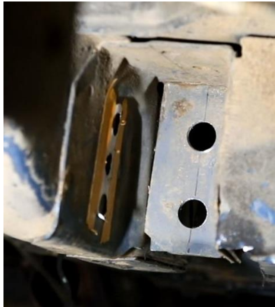
Figure 32 - Drill Plug Weld Holes
