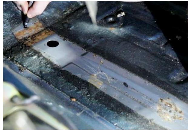
Figure 11 - Mark Front of Cut Area
