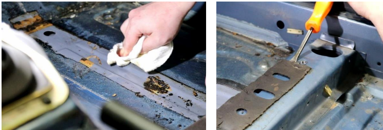
Figure 6 – Clean Cut Area and Remove Foam
