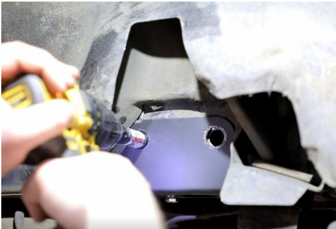
Figure 20 – Drill Frame Rail Holes
