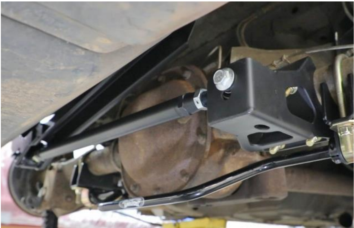
Figure 42 – Track Bar Installation
