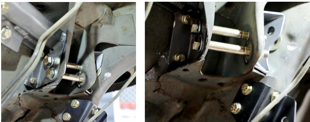
Figure 52 - Verify Installed Hardware
