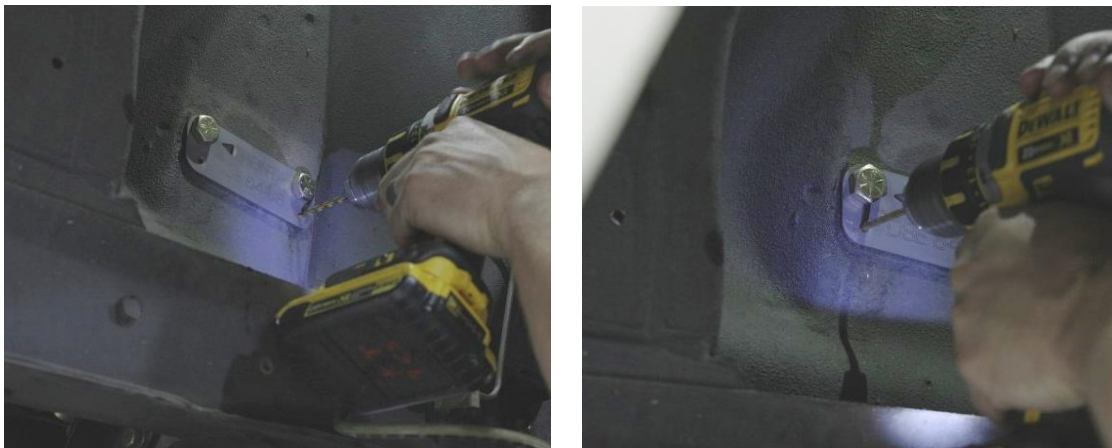
Figure 4 - Mark Drill Locations
