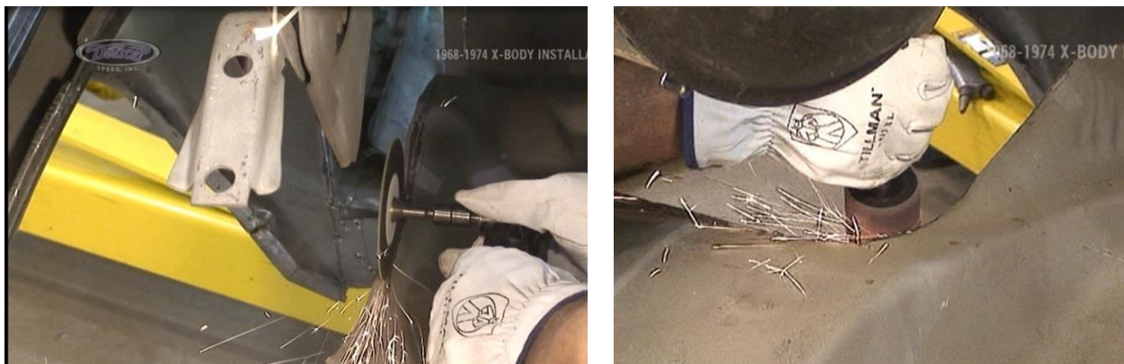
Figure 20 – Finish Cut and Grind Pre-Marked Lines
