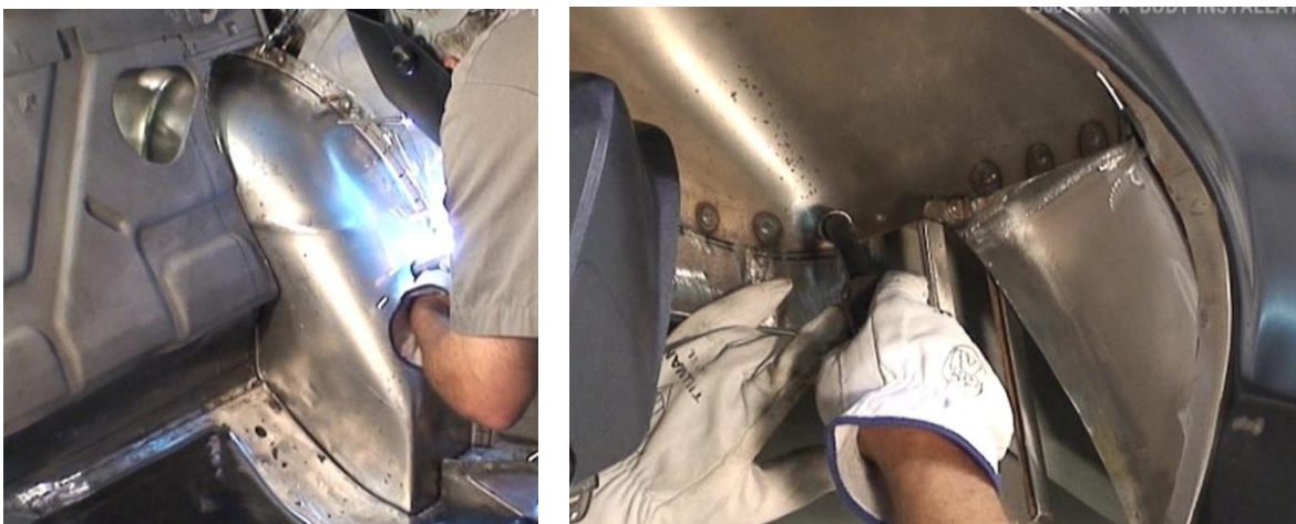
Figure 29 - Welding the Mini-Tub
