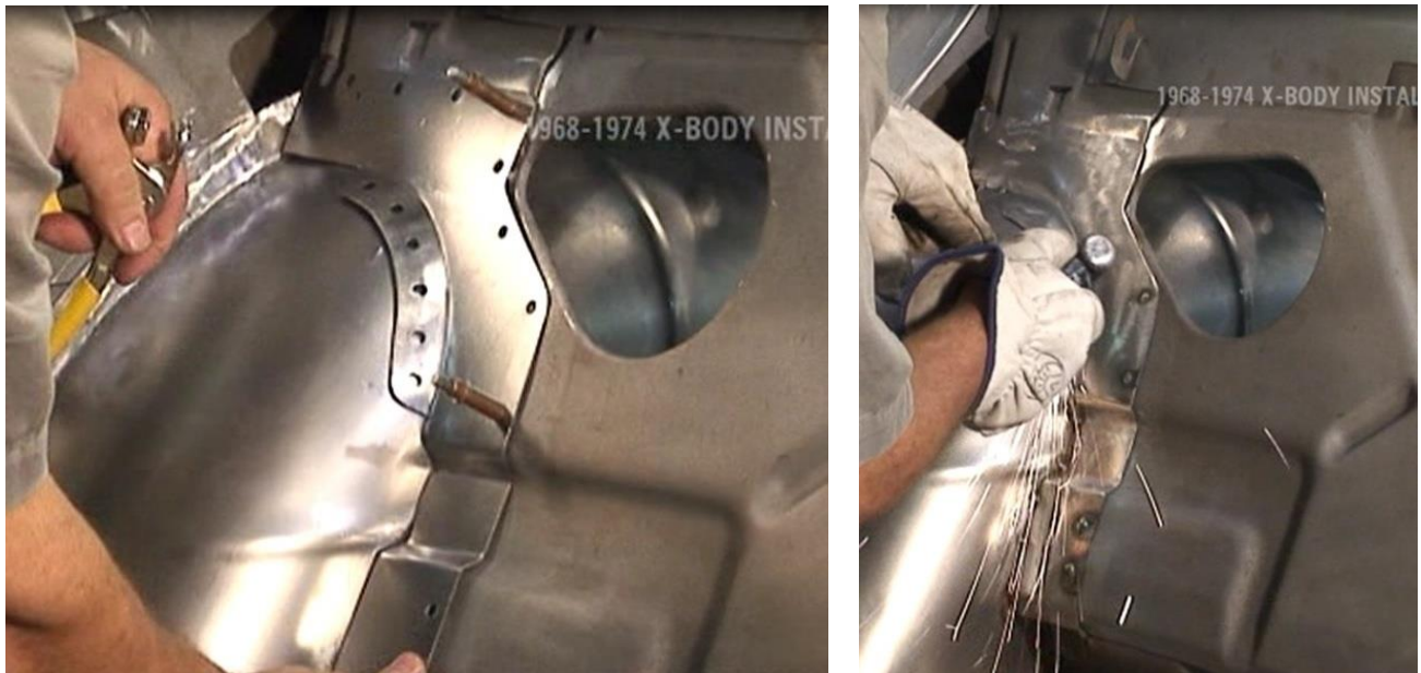
Figure 42 - Weld and Grind Seat Back Brace
