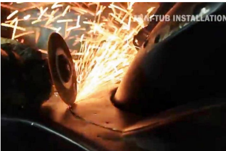
Figure 18 – Cutting the Trunk Floor
