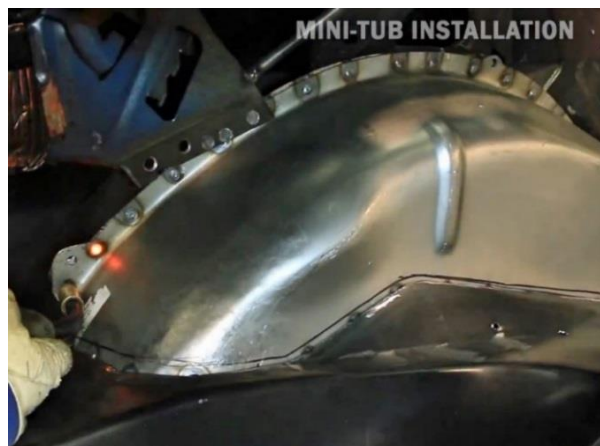
Figure 40 - Weld Detroit Speed Mini-Tub
