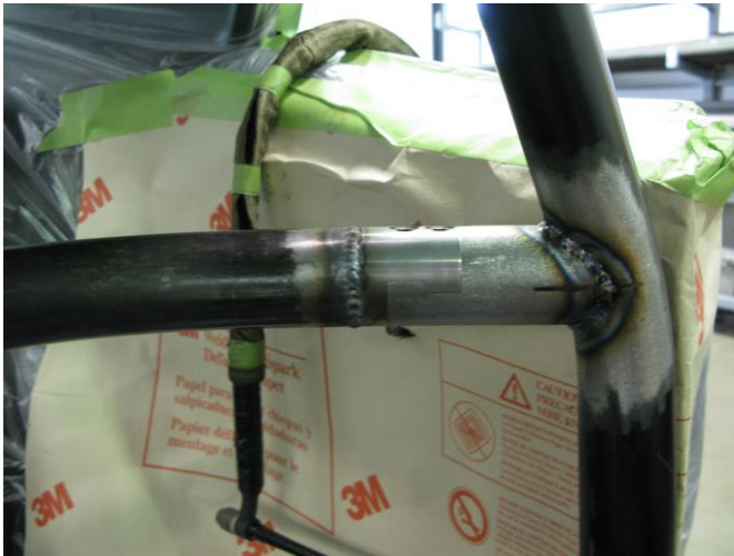
Figure 8 – (Finish Weld Cross Brace)
