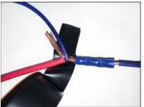
**Electrical Taping Bare Wires**
